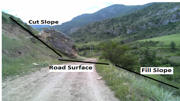
Figure 7) Forest road sample in the earth section
