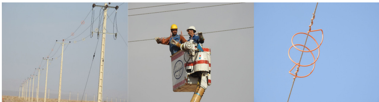
Figure 3) Installation of anti-collision spirals on power lines in the Abbas Abad Wildlife Refuge.
