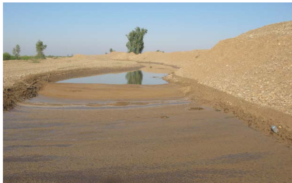
Figure 2) Embankments and infiltration pools in the Mosian FWS system
